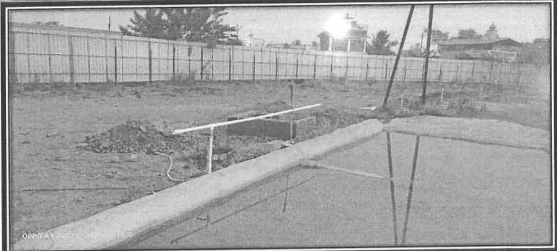
(Tyre Washing Point)
